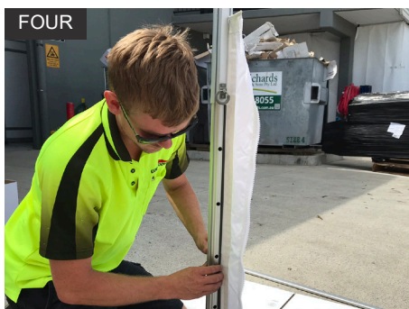
Press the Leg Rubber Inserts into the tracking on the Lower Leg of the Canopy. Repeat on other side.
