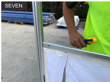
Insert the Wall Strip Keda into the Half Wall Bar. Insert the Half Wall Support Bar into the Tracking of the Upper Leg of the Canopy.
