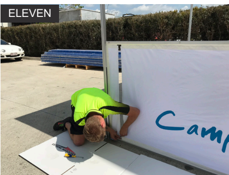
Zip the Wall Strip and the Half Wall Panel together.
