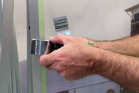
1. Position the Canopy Leg Connector in desired location and tighten until fitted.
