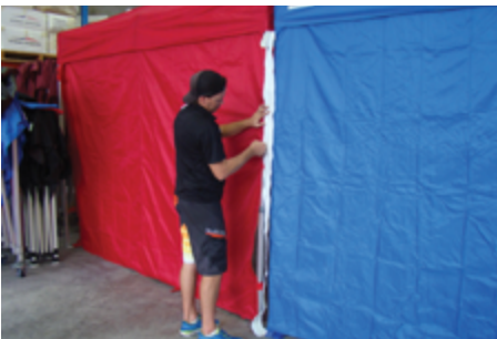
3. Attach rain gutter strip to tent wall.
