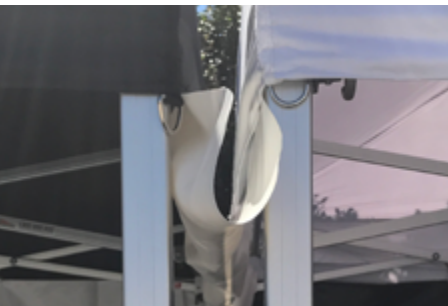
2. Put gutter hooks through eyelets in roof flap (face hooks inwards).
